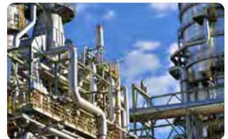
Kraftwerksbau | Power plant construction
