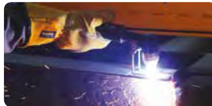
Manuelles Schneiden | Manual cutting
